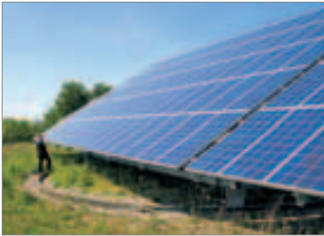
High-performance: : the “SunCarrier” has a module surface of 250 square metres and can supply power for up to 18 households.
